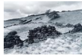
Stonewalls, Harworth Moor (19931096B)
