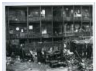
The "Golden Flats", South Side (20112418) Object identifier: 20112418 Name: The "Golden Flats", South Side
